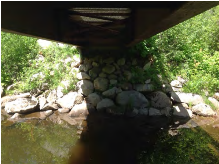
Left Bank Abutment when facing downstream
