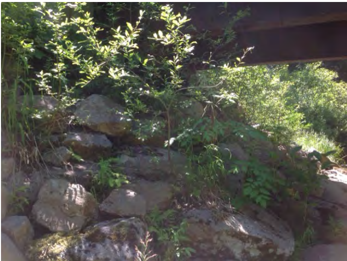
Right Bank Abutment when facing downstream
